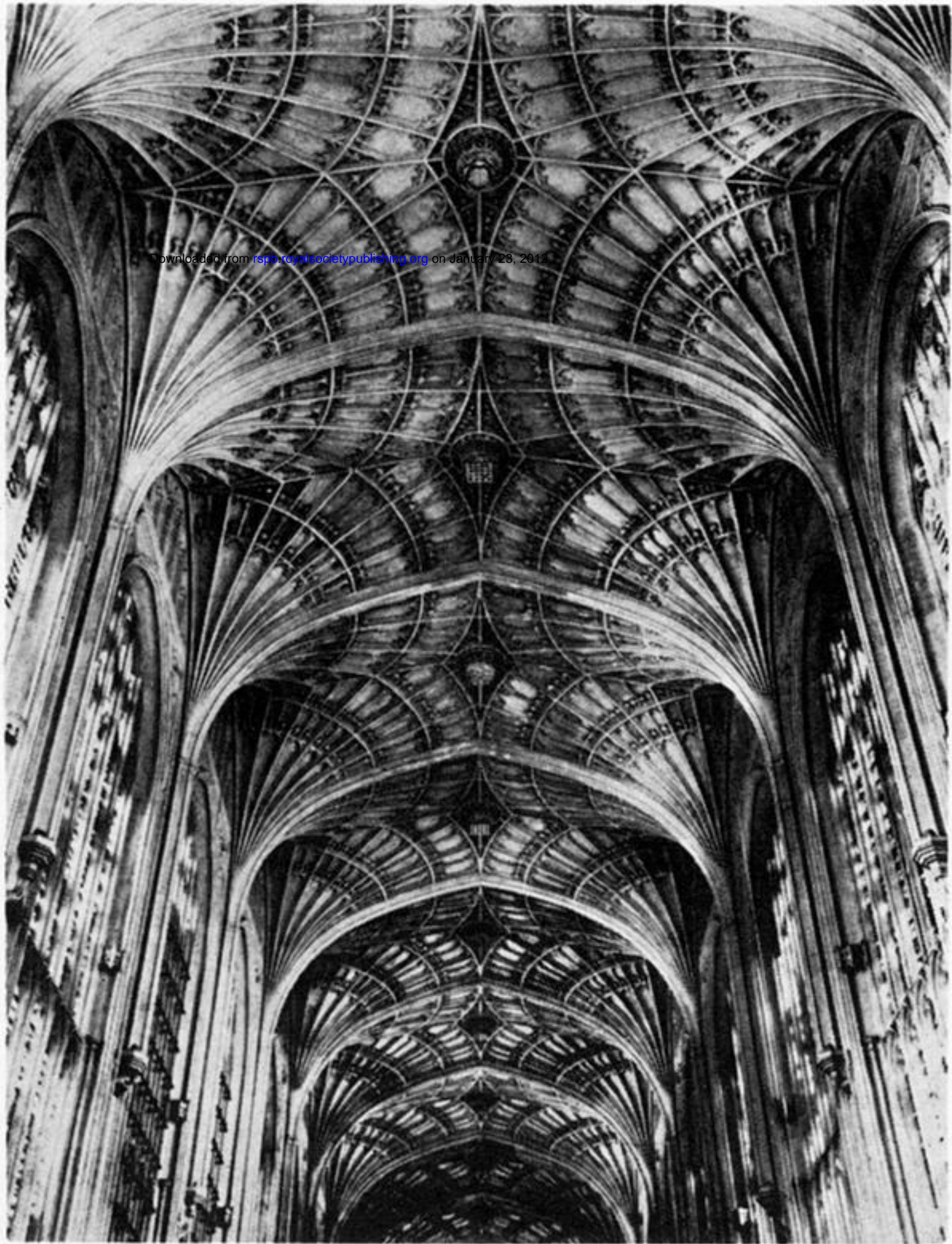
FIGURE 2. The ceiling of King's College Chapel.
