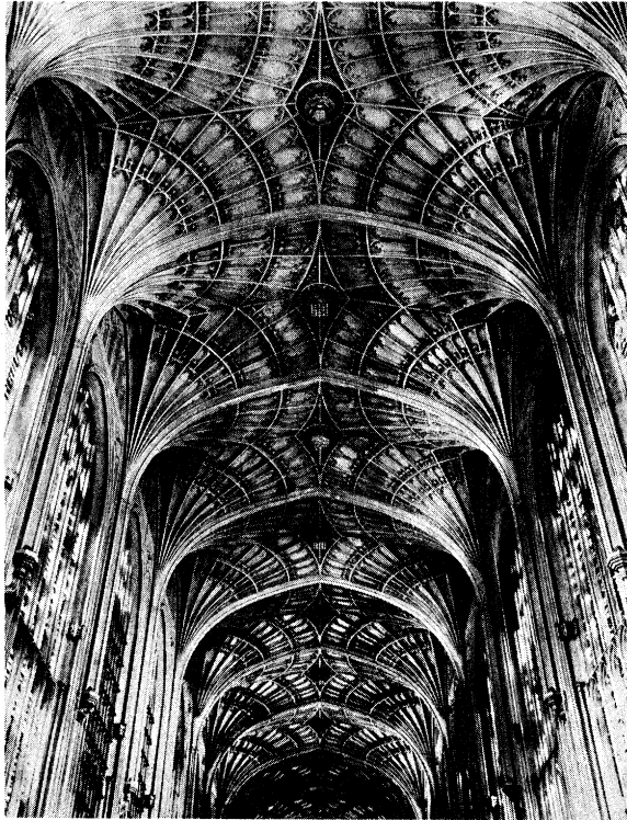
FIGURE 2. The ceiling of King's College Chapel.
